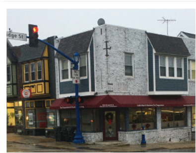
Office at 300 Bridge Street, Phoenixville
